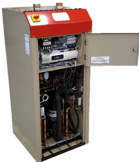
FRONT SERVICEABLE Severn unit shown with Service panel removed and control panel door open
